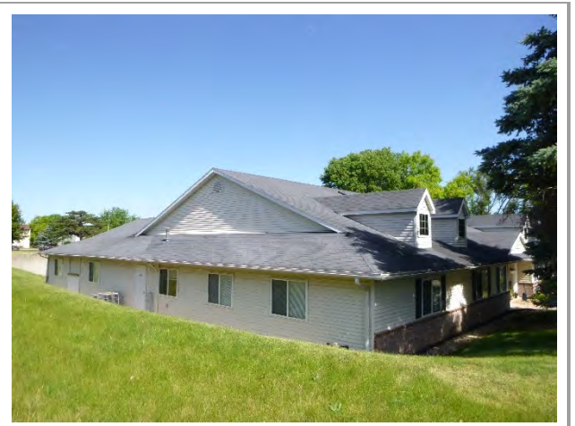
View of South and East Elevations
