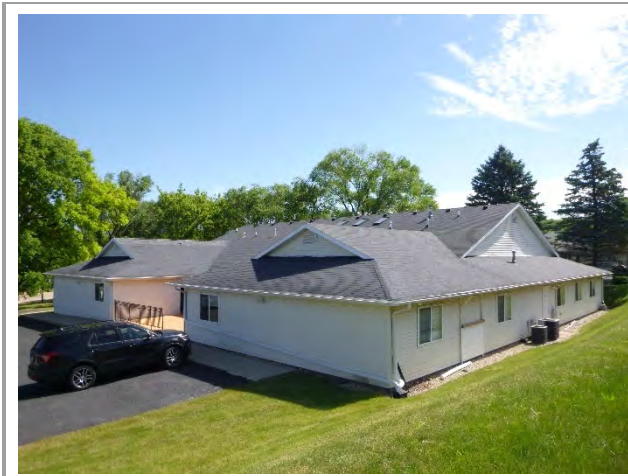
View of West and South Elevations
