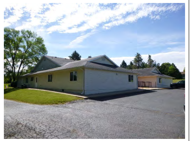
View of North and West Elevations
