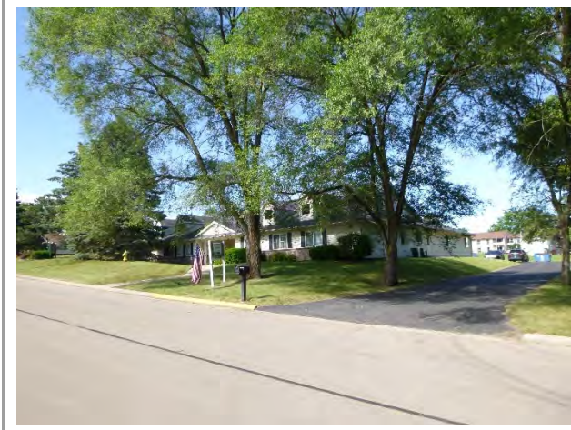
View of East and North Elevations
